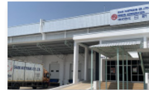
Dangerous goods warehouse
